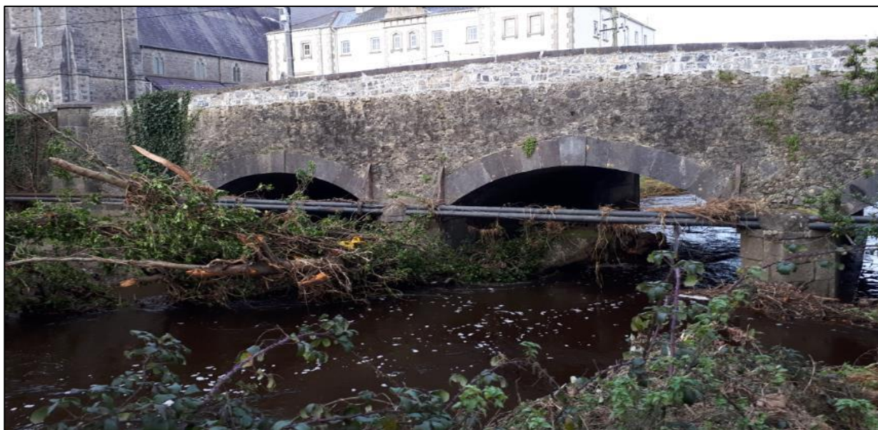
Figure 6-14: Blockage at Convent bridge
